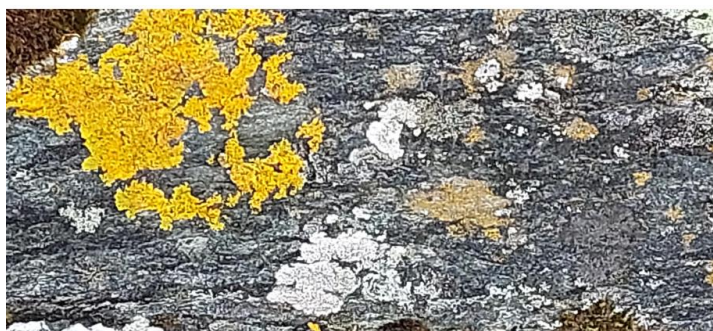
Figur 8 Messinglav, observert under befaring 25.03.2022.
