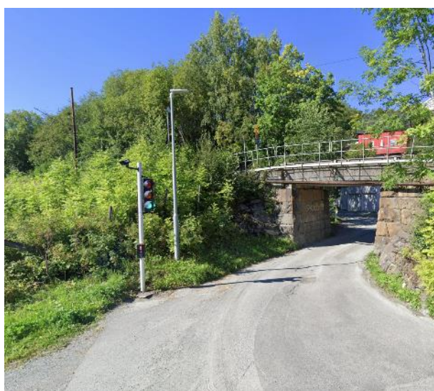
Figur 14: Signalregulert undergang under jernbanen.
