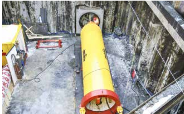
Tunnelering under E39.
